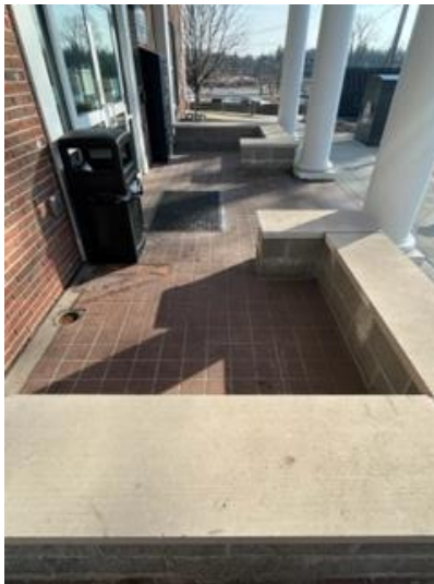
Side view of back entryway
