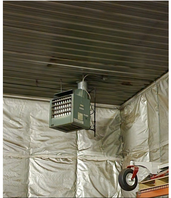
North Unit Heater Parking Barn
